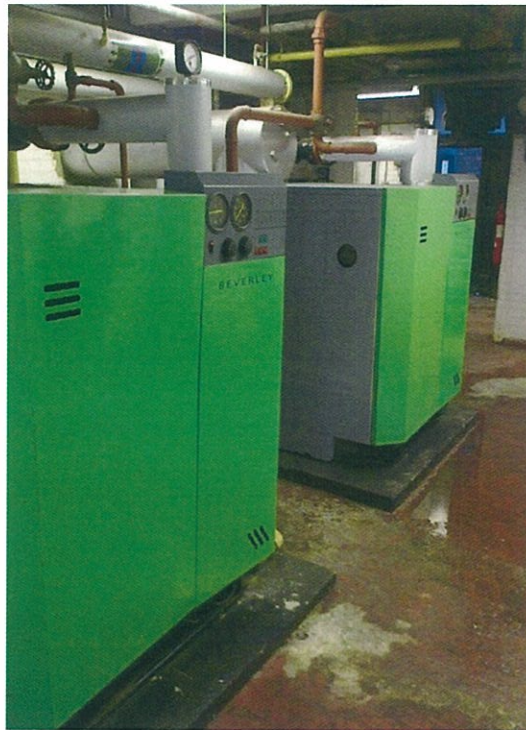
Photo 19 Basement heating boilers, water ingress
