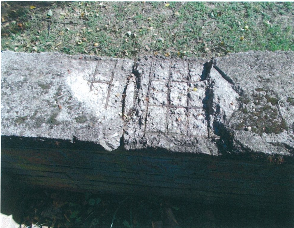
Photo 4 Example Condition of Concrete Copings
