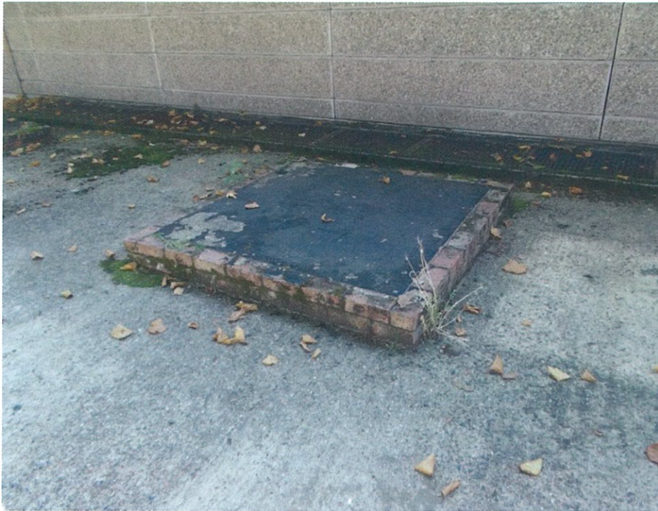
Photo 5 Basement Penetrations to North Hard Standing
