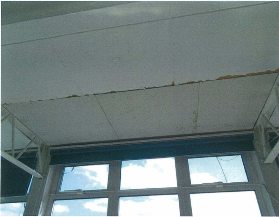
Photo 15 Failing Ceiling Boards
