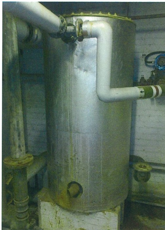
Photo 19 Basement heating boilers, water ingress
