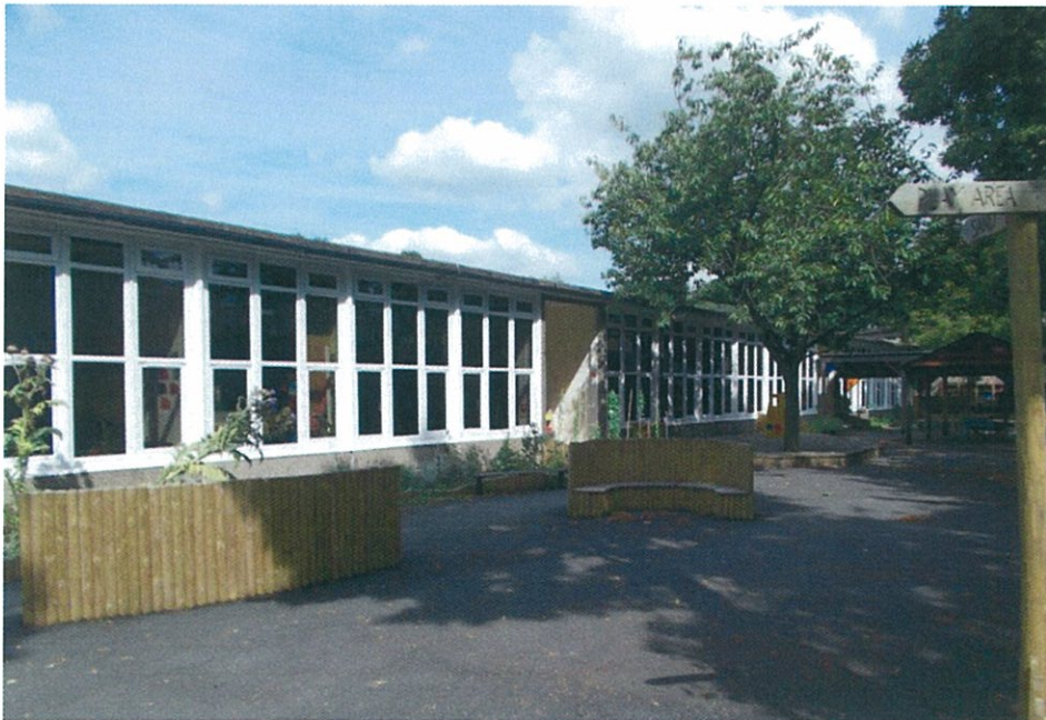
Photo 10 General View of South Wing
