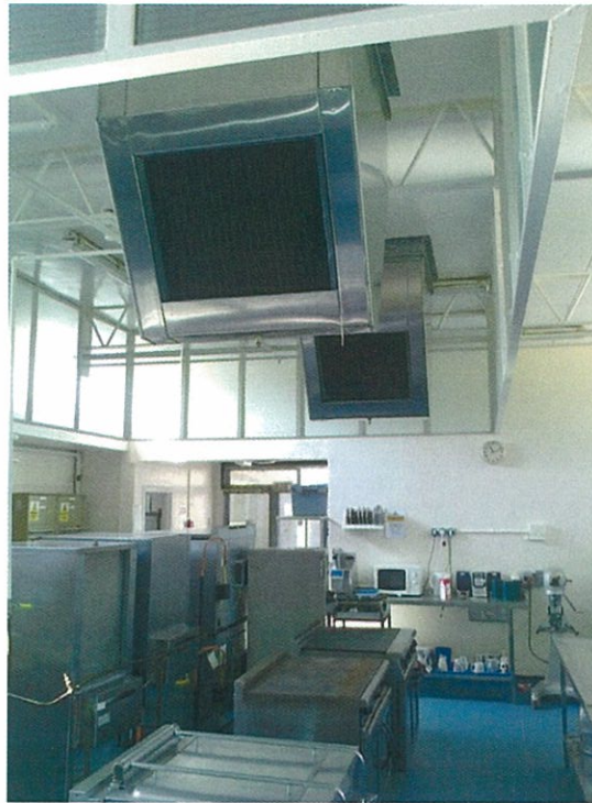
Photo 25 Main kitchen, extract ventilation to all electrical catering equipment
