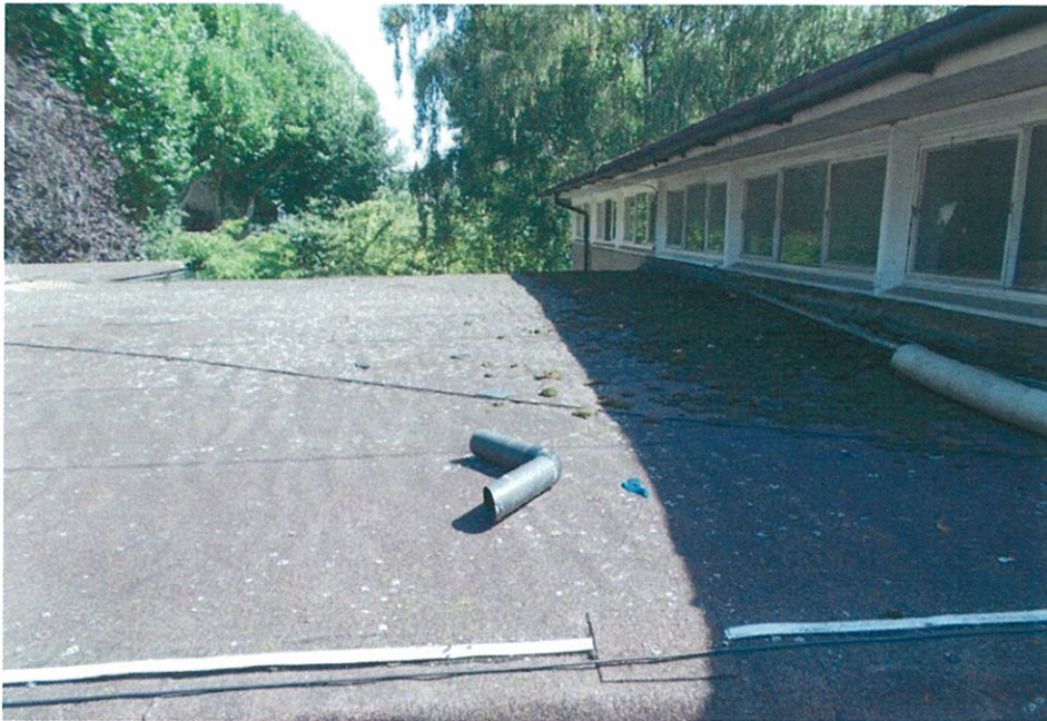
Photo 6 Example Condition of Roof Covering
