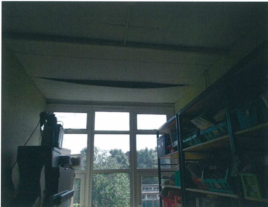
Photo 15 Failing Ceiling Boards
