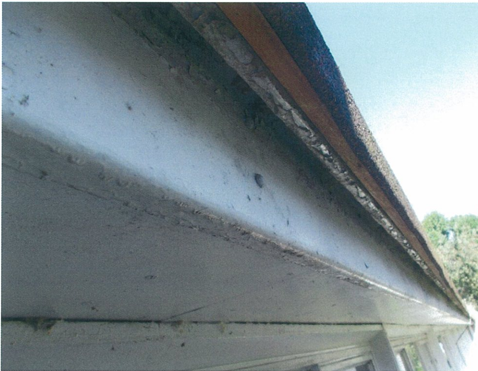
Photo 3 Example Condition of Eaves
