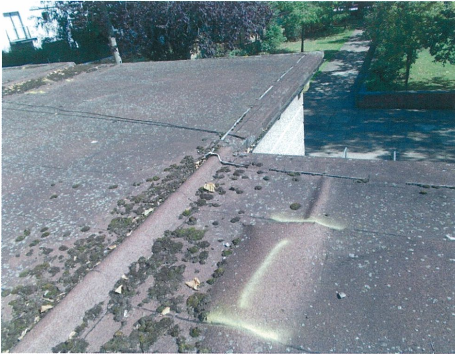
Photo 7 Example Condition of Roof Covering
