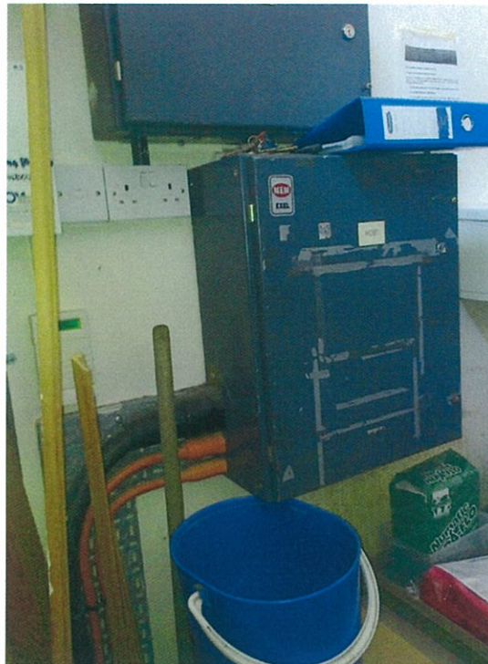
Photo 21 Local electrical distribution, in cleaner's cupboard
